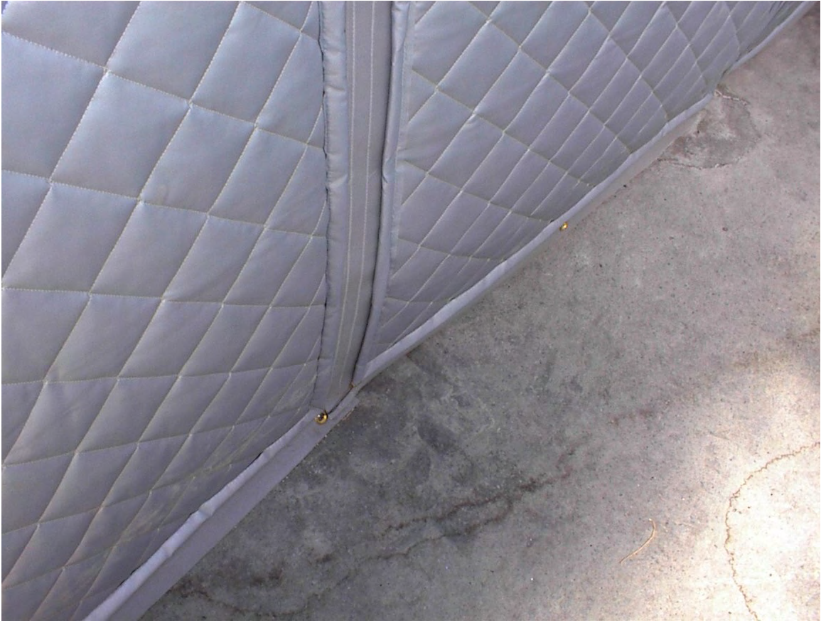
Figure 7 Panels must touch the ground; some curl is okay.
